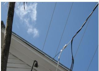
Wedge clamps are mechanical holding devices used for strain relief in service applications.
